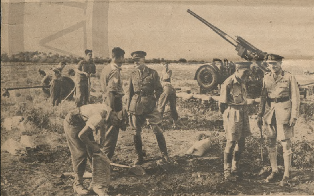
Work on the defences has already started and the G.O.C.-in-C. inspects the results.
