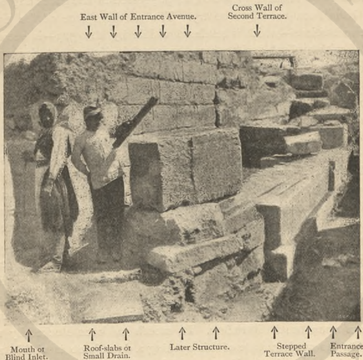
FIG. 22.—SECTION OF NORTH ENTRANCE WAY SHOWING EAST WALL AND STEPPED WALL OF TERRACES.
